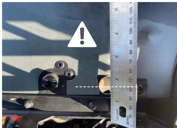
Fig. 3: Second mark for drill hole
